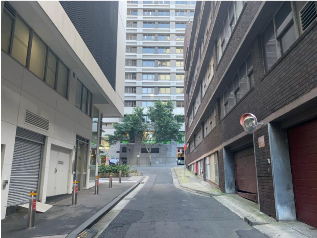
Figure 7: Alberta Street, view facing north showing the existing tower
